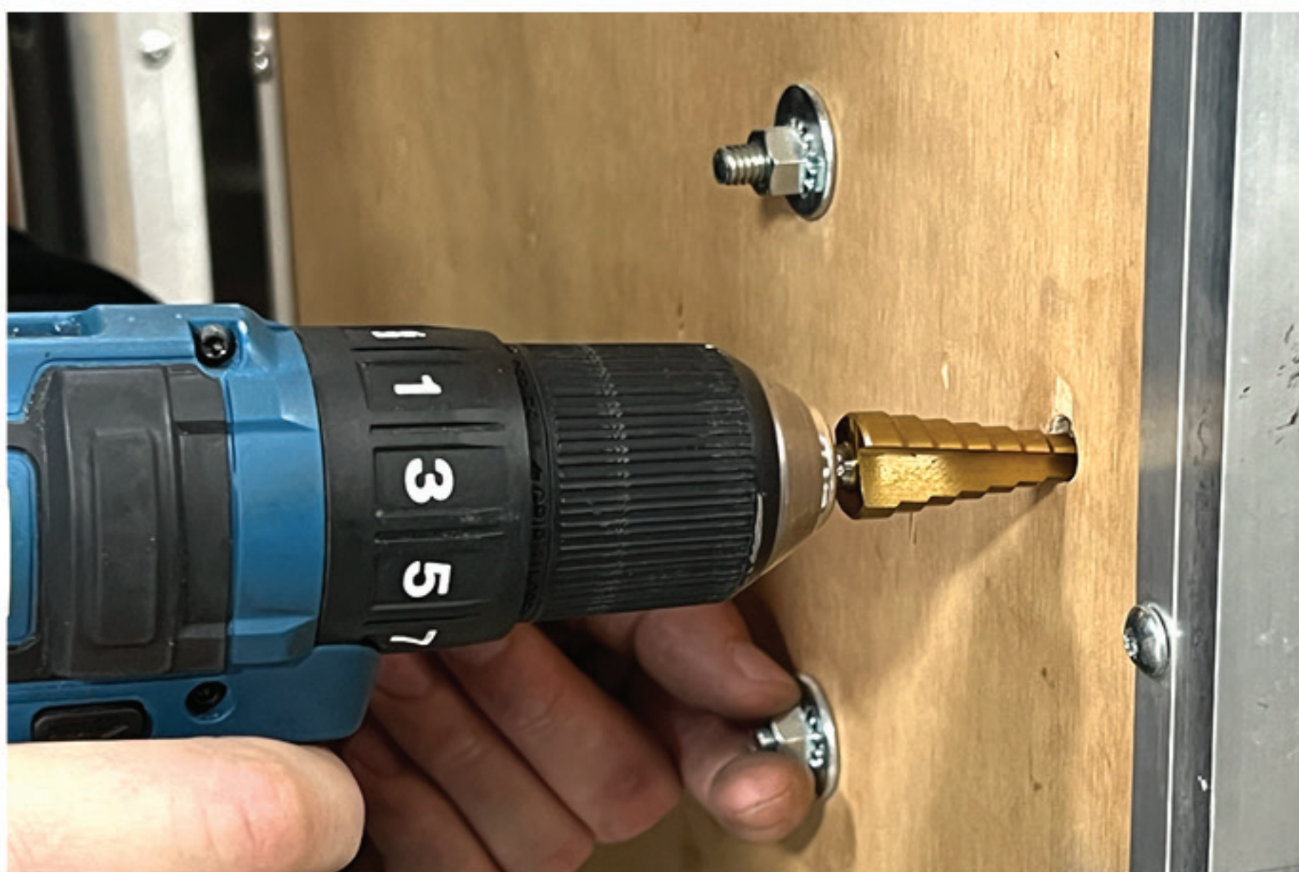
Do the same on the inside of the door using the step bit.
