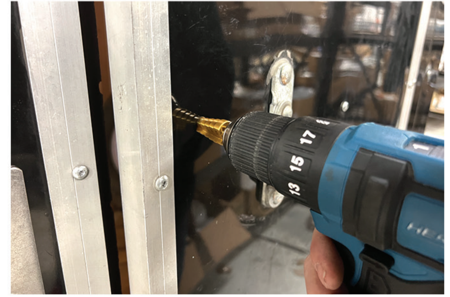
Using a step bit clean the hole edges on the outside of the door.
