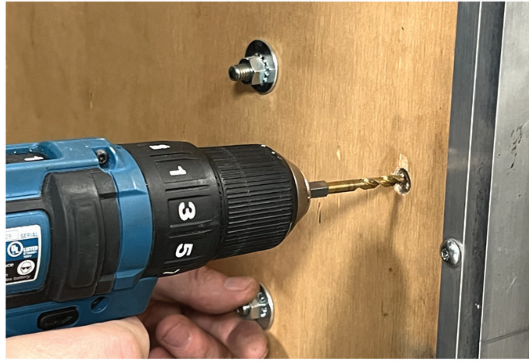
Drill on the marked spot using a 7/16" drill bit. Drill the hole straight and level until it reaches the outside of the door.
