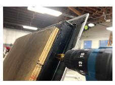
Enlarge the hole in the ramp door using the step bit to fit the bolt. Refrain from making the opening too large. You can always return to make it larger if needed.
