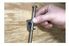
Secure the Lock Pin holder to the interior wall with the provided screw.
