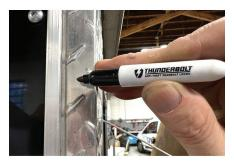
Locate the spot on the outside edge of the trailer where the anchor will be installed. The spot should be as flat as possible and fit the diameter of the anchor.
