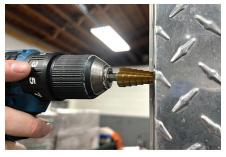
Open the hole on the outside of the trailer to 11/16" using the provided step bit from the installation kit. The hole will then fit the Tap also included in the kit.
